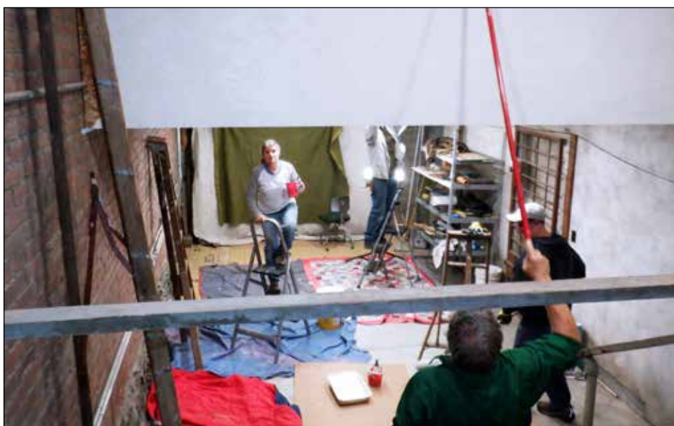
Volunteers paint the ceiling and walls
